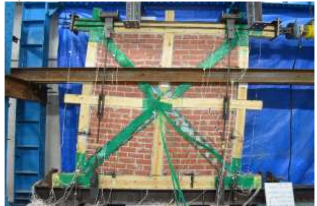
Figure 15: Damages of the AFRP sheets on the front side (S5)
