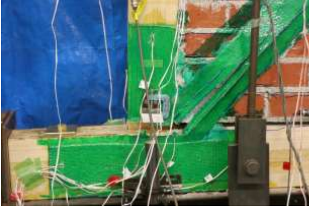
Figure 17: Fracture of the AFRP sheet on the front side of the bottom left connection (S5)
