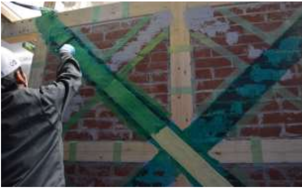
Figure 6: Application of the AFRP sheet on S3 and S4, respectively [7]
