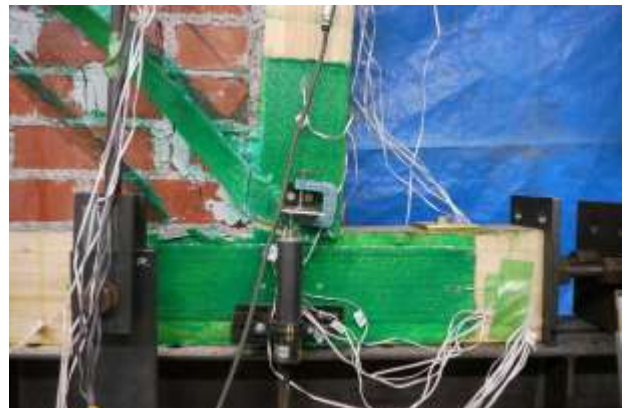
Figure 16: Fracture of the AFRP sheet on the front side of the bottom right connection (S5)
