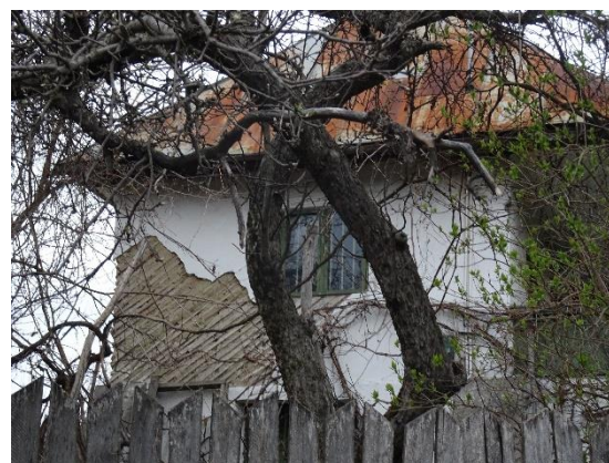
Figure 10: Detail of traditional house with timber skeleton and strips applied at 45° and clay plaster (Type 2) from Mustățești, Argeș county;
