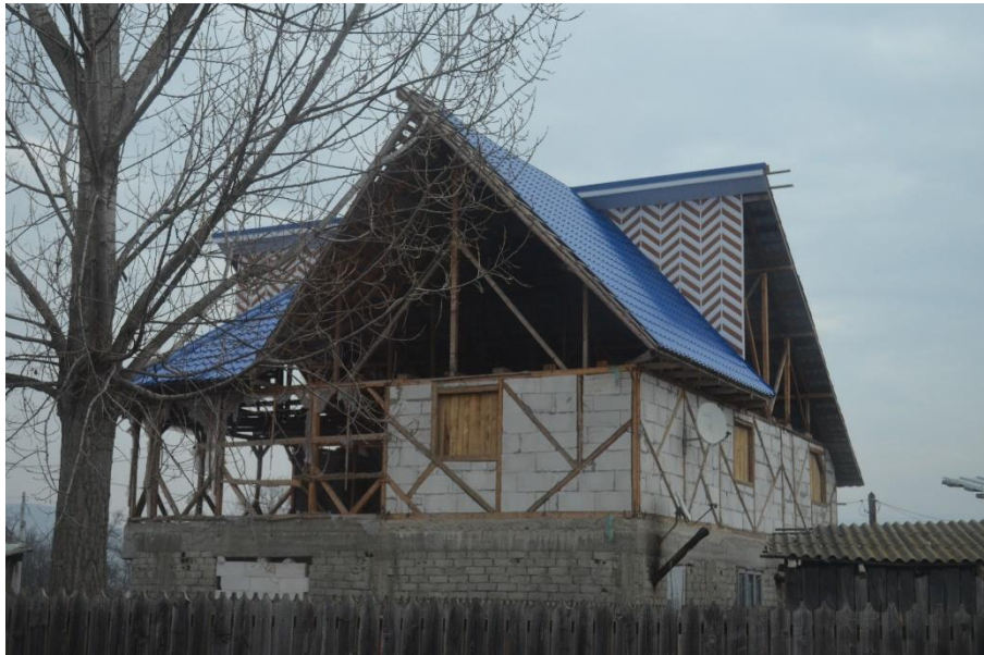
Figure 19: Building with timber skeleton and AAC (autoclaved aerated concrete) masonry infill (Type 5), from Viperesti, Buzau county
