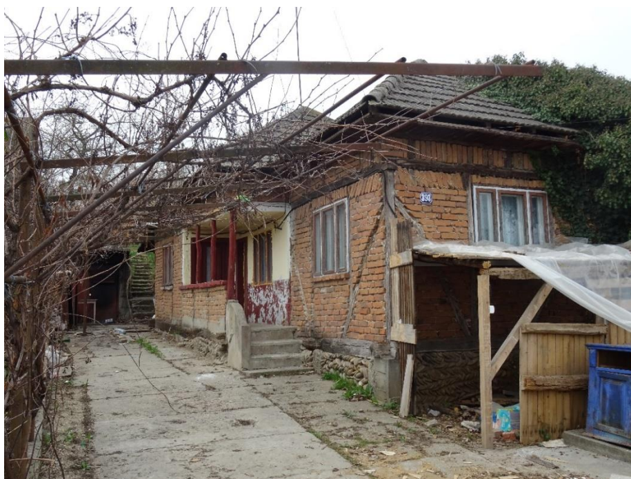
Figure 7: Traditional house with timber skeleton and brick masonry infill (Type 1) from Teiș village, Dâmbovița county
