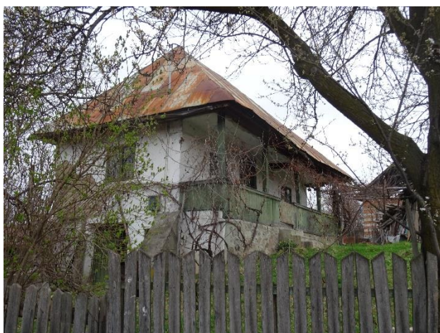
Figure 9: Traditional house with timber skeleton and strips applied at 45° and clay plaster (Type 2) from Mustățești, Argeș county;
