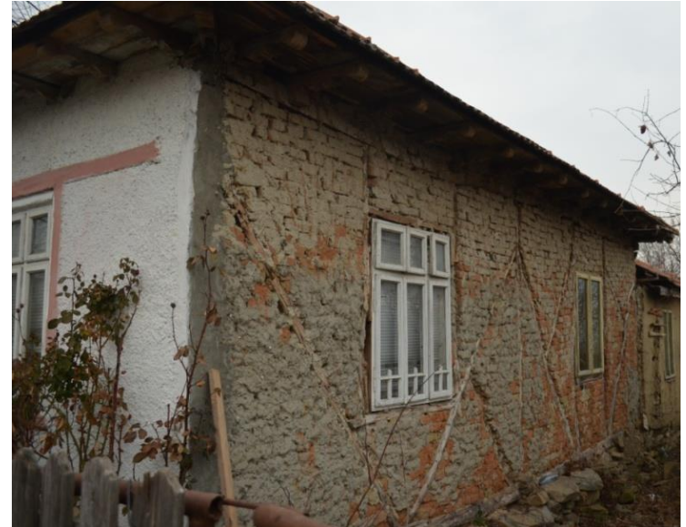
Specimen S1 (from type 1) - timber and brick masonry infill structure: 1 – inferior stringer; 2- column; 3 – bracing; 4 – superior stringer; 5 – masonry infill; 6 – iron nails and cross – halving connections of timber elements (columns and strings)
