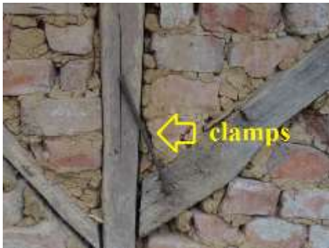
Figure 16: Clamps used for timber elements connections
