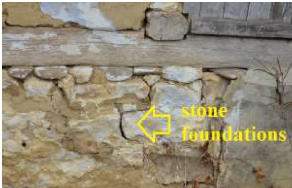
Figure 12: Stone foundation specific for the traditional buildings, the old ones
