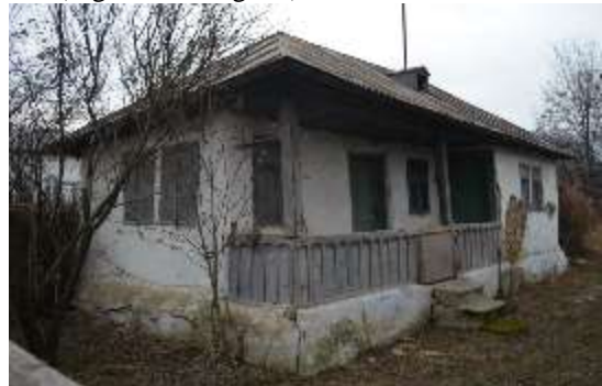
Figure 10: Building with timber and wattle and daub infill structure, from Viperesti commune, Romania, built in around 1910-1920 – main façade
