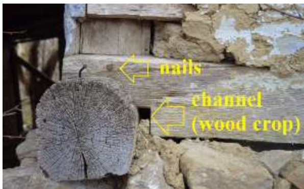
Figure 17: Nails and cross-halving for timber elements connection
