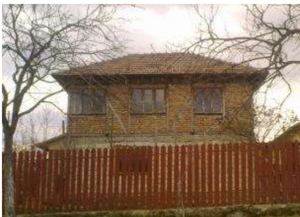
Figure 2: Traditional infilled timber frame house from Buzau county [4]
