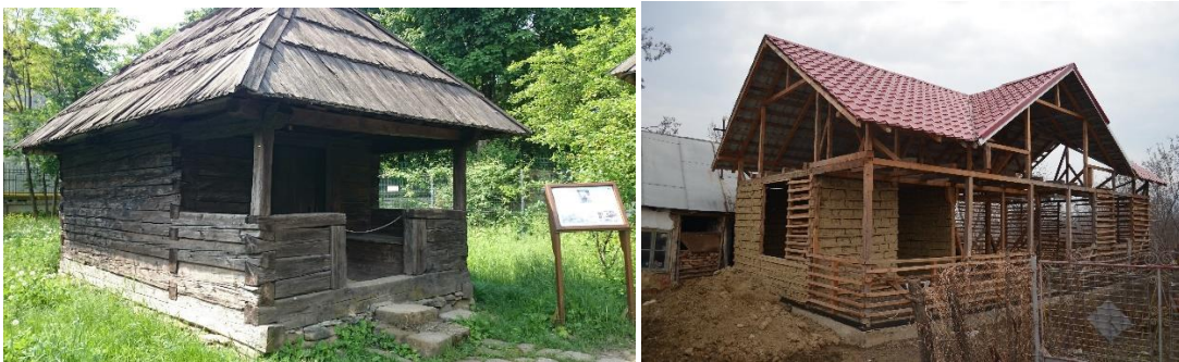
Figure 1: The adaptation of house structure, due to lack of timber: left [2] is typical for mountain areas (where timber is easy to find) and right is in a hill area (where timber is not so cheap)
