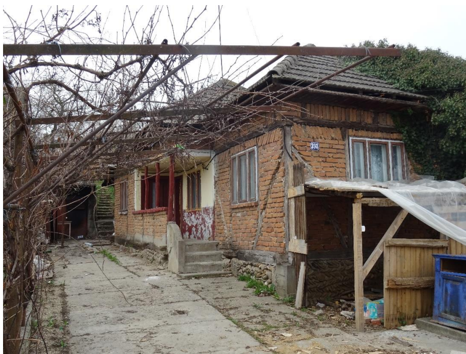
Figure 7: Traditional house with timber skeleton and brick masonry infill (Type 1) from Teiș village, Dâmbovița county
