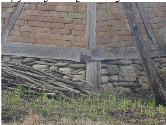
Figure 15: The foundations are made only from stone (river rocks)
