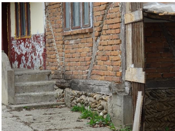
a. The foundations are made only from stone (river rocks)
