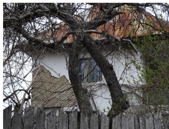
Figure 10: Detail of traditional house with timber skeleton and strips applied at 45° and clay plaster (Type 2) from Mustățești, Argeș county;
