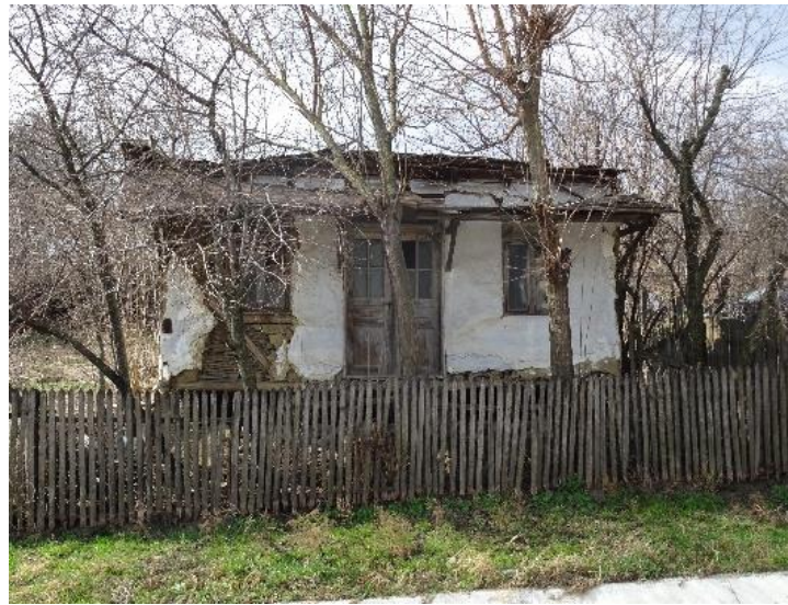
Figure 11: Traditional house with timber skeleton and wattle and daub (Type 3 – ”grădele”) from Băbeni, Vrancea county
