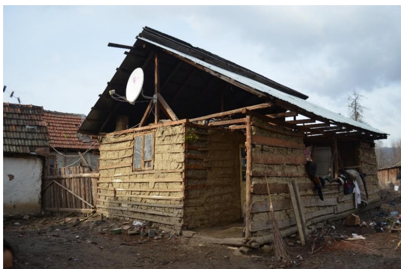
Figure 13: Building with timber and earth with straw infill structure (Type 4), from Viperești, Buzău county
