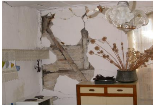
FIG. 13. GENERAL 3-DIMENSIONAL VIEW OF THE TRADITIONAL WOOD FRAME, REGIONAL, CONSTRUCTION OF THE ISLAND OF LEFKADA (GREECE).
